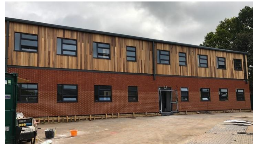
Euston Street Stores 179.9 kWp PV system
