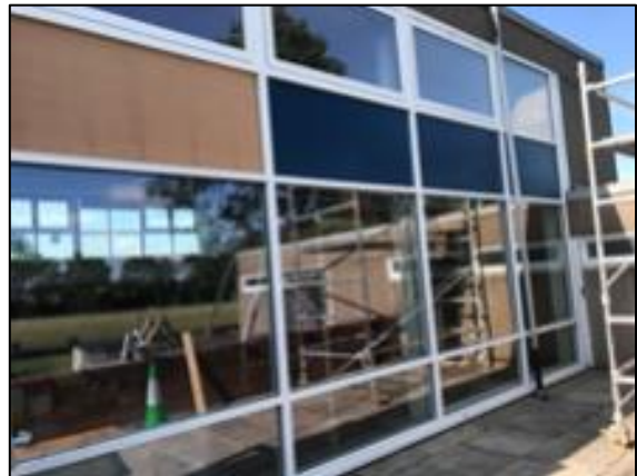
Newly installed windows
